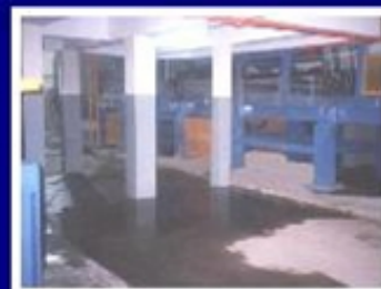
View below mezzanine waste tipping floor
